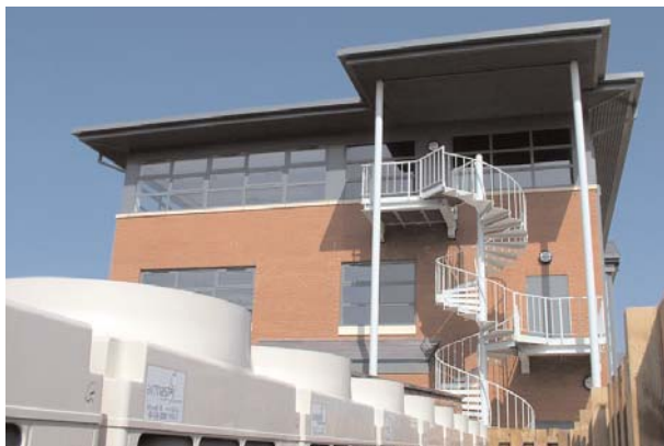
The condenser farms do not disturb the neighbours
