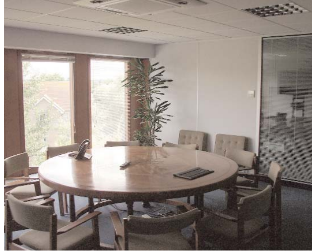
A board room with Toshiba ducted units and the original fixtures and fittings preserved
