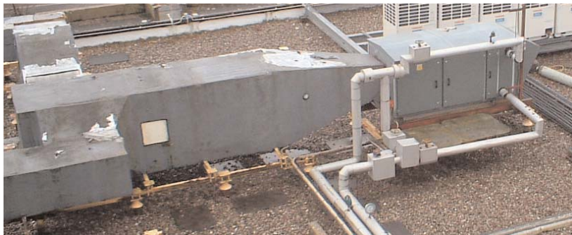
Old systems had to be taken away
