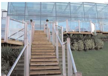
The extent of the glazing means high heat losses and gains
