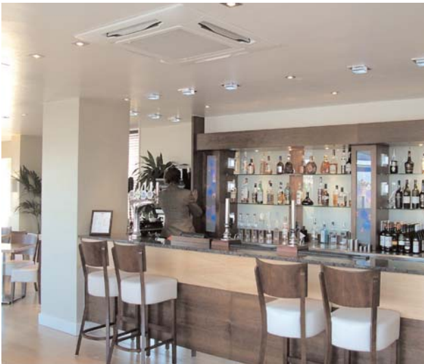
The four-way cassettes work well in the bar
