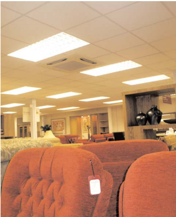
Air conditioning enables the store to use its former warehouse as sales space
