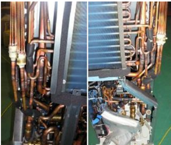
Pipe work after
